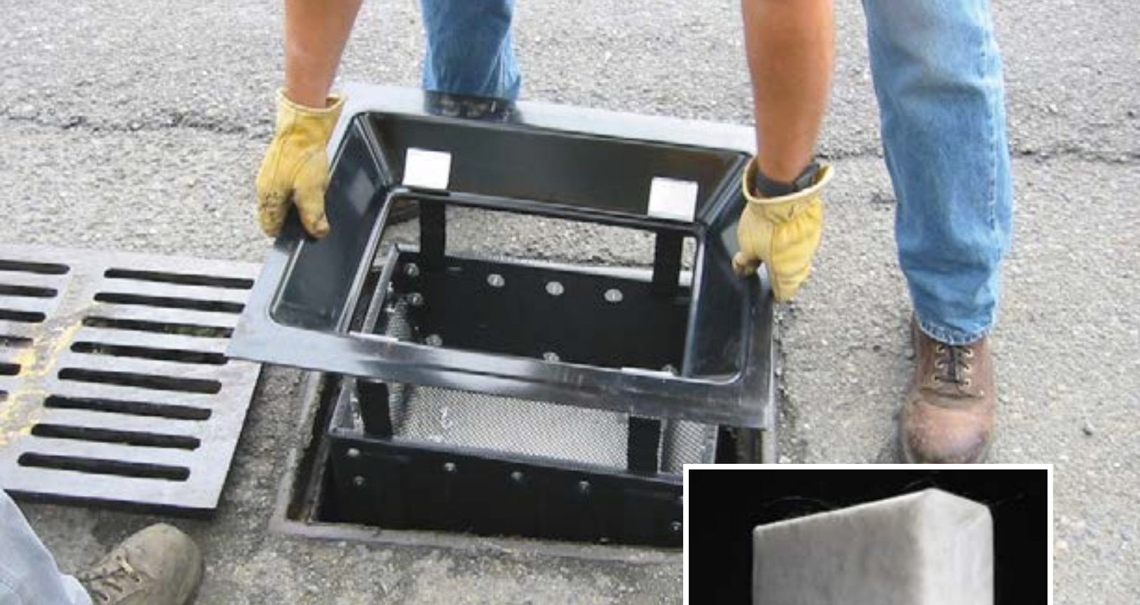
Smart Pak® Cartridge insert filled with Smart Sponge® Media
